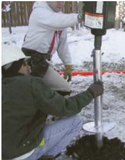
Figure 3. A bobcat or small excavator with an auger attachment turns the lead section into the ground. Additional sections are added until the pier encounters enough resistance to stall the motor. The soils common to the author's area usually take one lead section and one extension.
