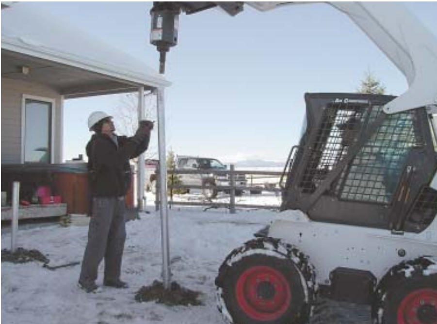
Figure 3. A bobcat or small excavator with an auger attachment turns the lead section into the ground. Additional sections are added until the pier encounters enough resistance to stall the motor. The soils common to the author's area usually take one lead section and one extension.
