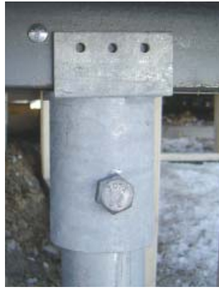
Figure 4. Once all the piers are installed, a site level is used to cut them to uniform height. U-shaped saddles bolted to the piers (above) receive the beams that support the floor system (left).
