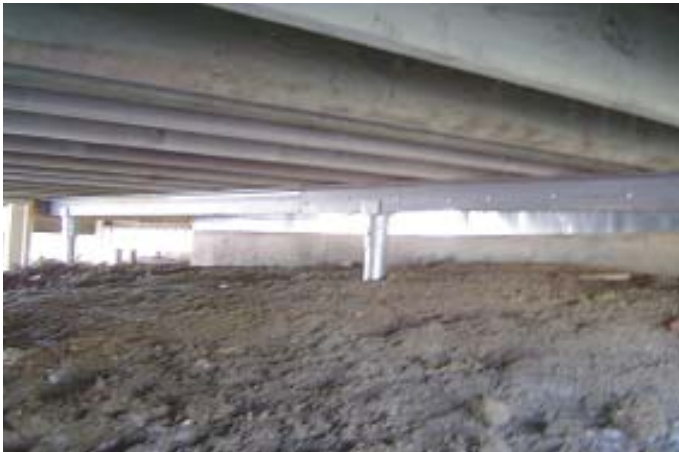
Figure 4. Once all the piers are installed, a site level is used to cut them to uniform height. U-shaped saddles bolted to the piers (above) receive the beams that support the floor system (left).
